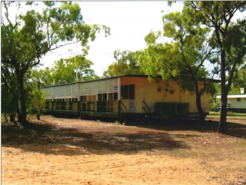
Mornington Island State School, High School block
